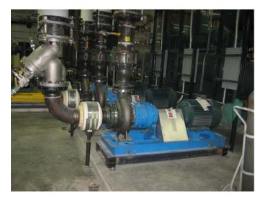
ACKETED BEARINGS SUPPORT JACKETED CASING JACKETED BRACKET
